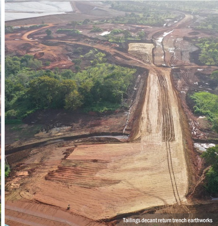
Tailings storage facility
