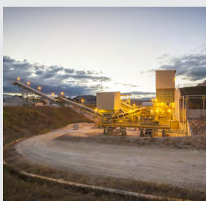
San Jose Mine crushing circuit
