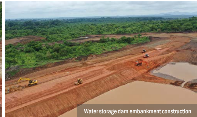
Water storage dam embankment construction
