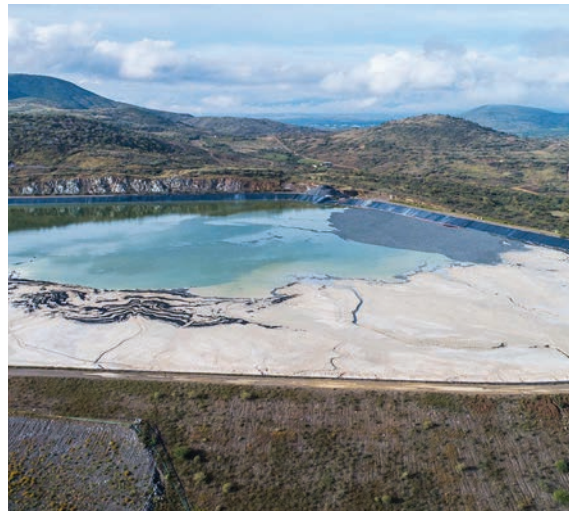
San Jose tailings pond
