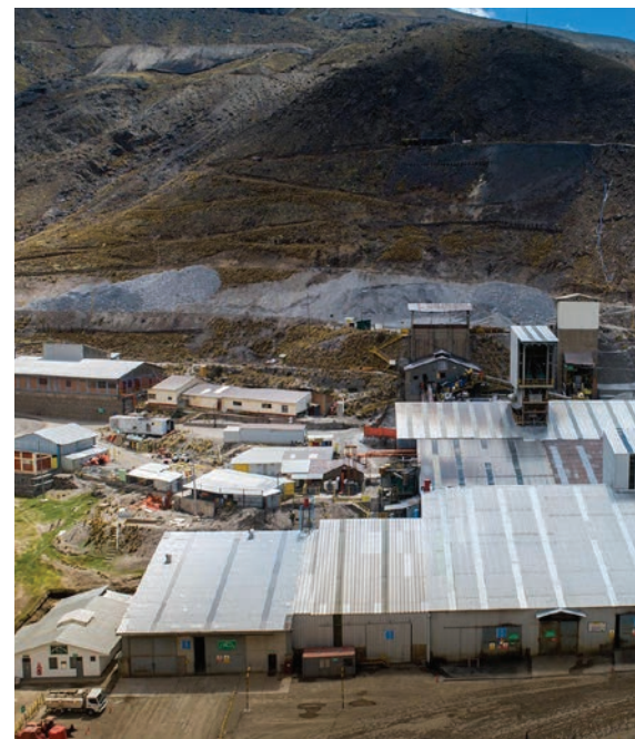
Caylloma Mine facilities
