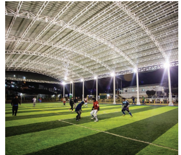
Sport and activities court in Caylloma Mine
