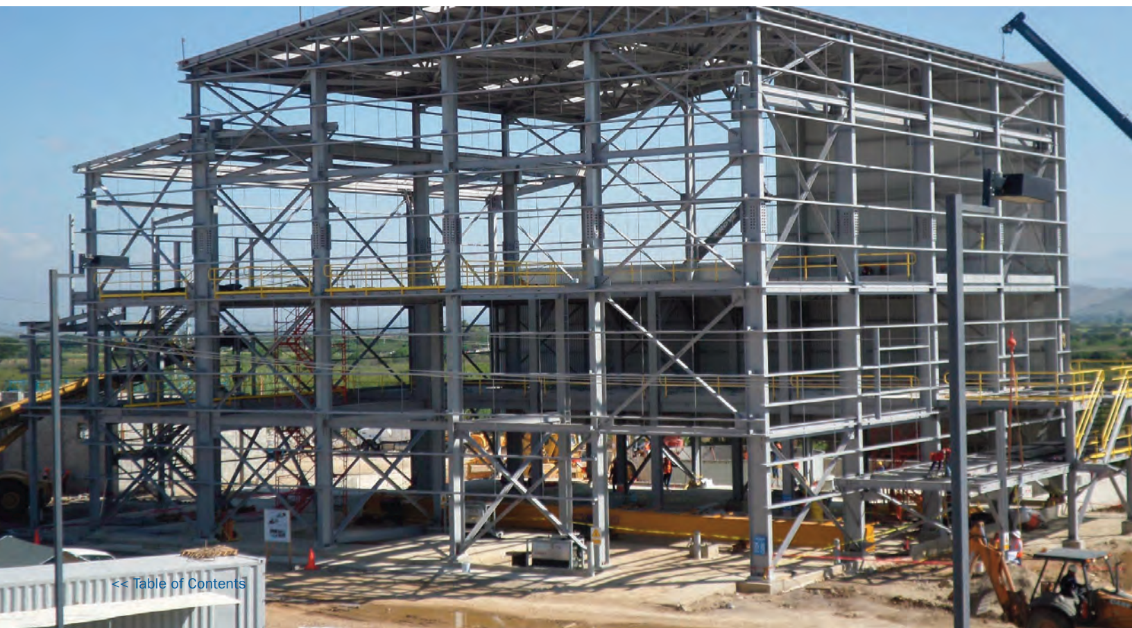
Dry stack tailings filter facility under construction
